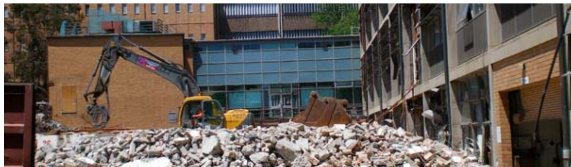
Demolition of the old Biochemistry building at the University of Melbourne.
